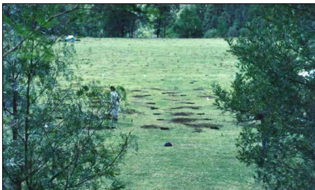
The post holes ready to build Kodoji, Gorricks Run, 1996 Photo: Caroline Josephs
