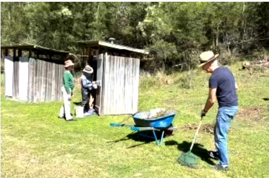
Maintenance of the toilet doors.
