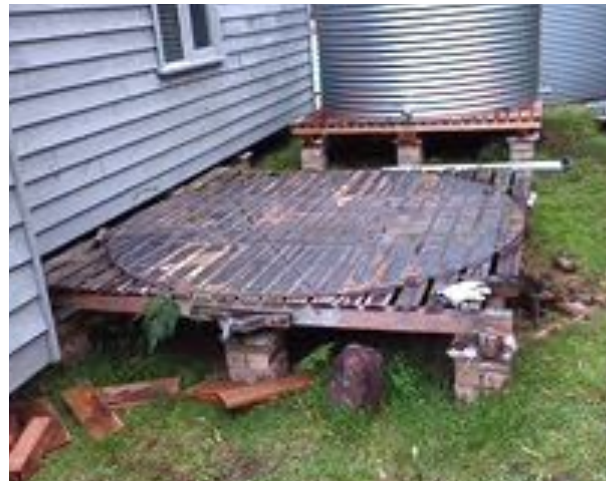
The old tank stand was replaced
